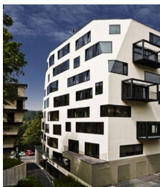
Triplex - residential building, Karlovy Vary
