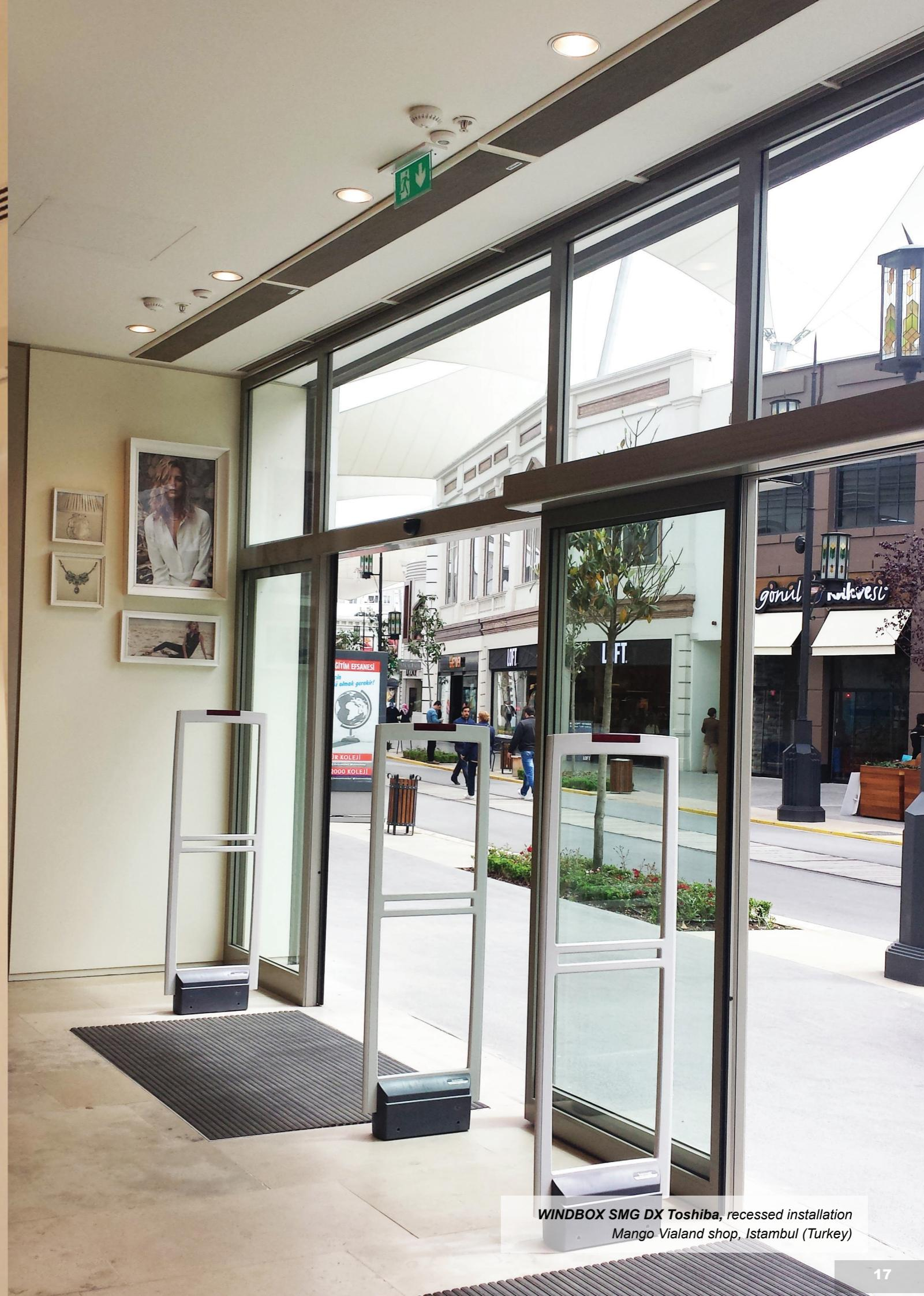
WINDBOX SMG DX Toshiba, recessed installation
