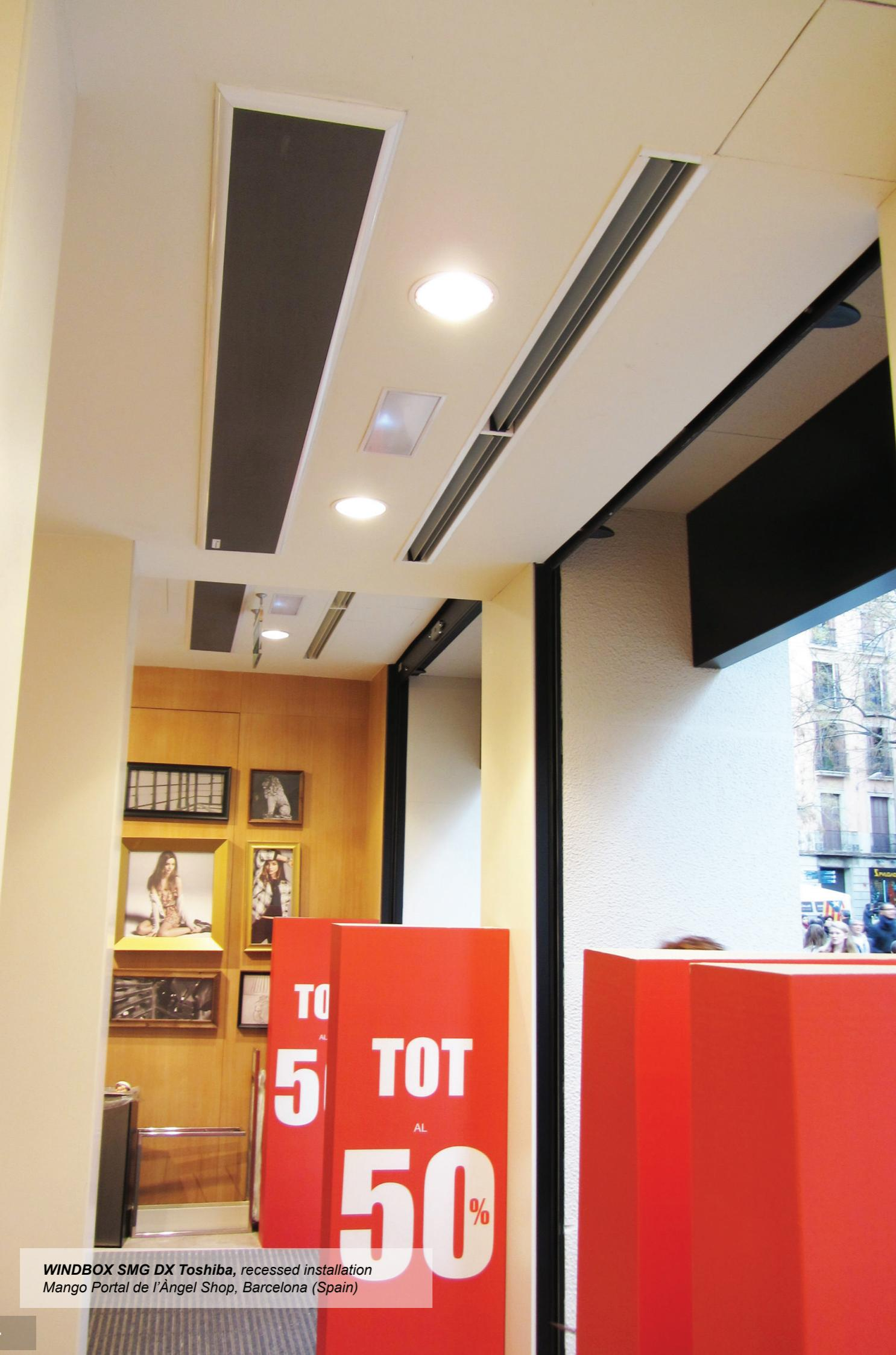
**WINDBOX SMG DX** Toshiba, recessed installation
